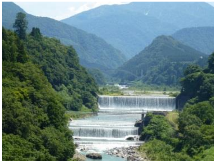
Hongu Sabo Dam ; National Registered Tangible Cultural Properties
