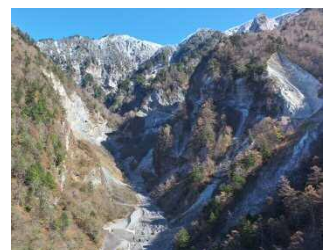
Series of Sabo dams in Shiratani Valley
