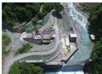
Kuronagi-River No.2 Downstream Sabo Dam (under construction)
