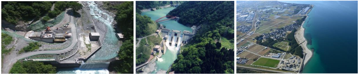
Kuronagi-River No.2 Downstream Sabo Dam (under construction)
