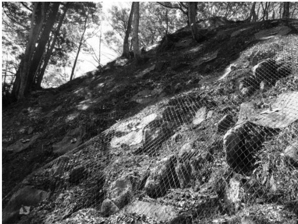
**Photo 1.** An example of slope stability works used by high tensile strength steel net.
