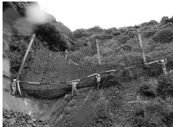
**Photo 2.** An example of capture of debris by flexible debris flow barrier.
