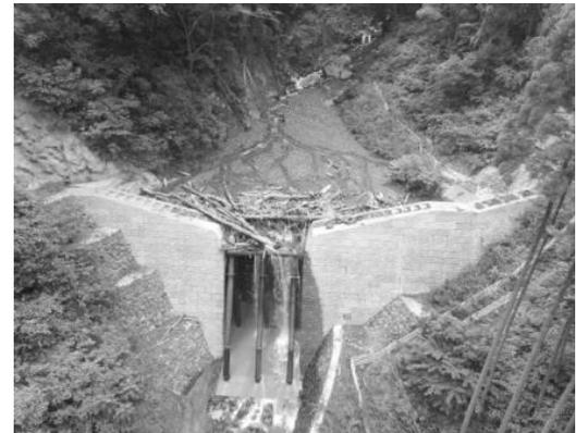
**Photo 1** Example of sediment control dam to catch debris flow and driftwood (Kirishima City, Kagoshima Prefecture)
