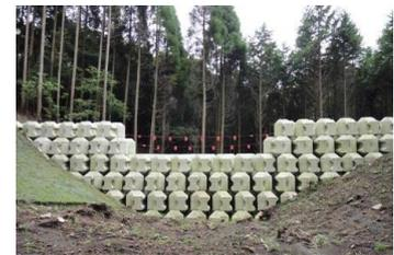
**Fig.2** Image of developing concrete block masonry sabo dams (Mt.Shinmoedake in 2011)
