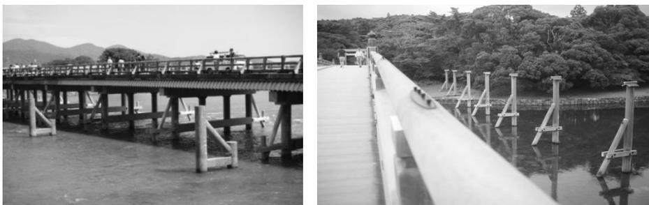
**Photo 1** Traditional Japanese technique to protect historical bridges using stakes (right: Togetsu Bridge, Arashi-yama, Kyoto; left: Uji Bridge, at the Ise shrine, Mie).
