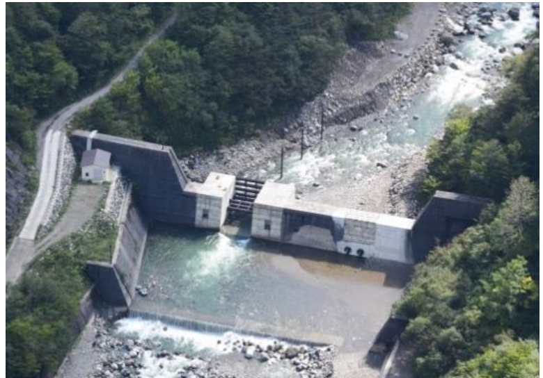
Myo-Jyu Sabo Dam with movable “shutter” Gate SABO Dam
