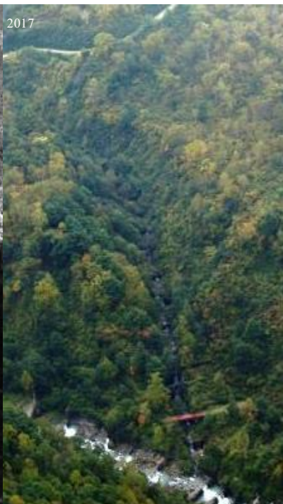
Dorodani Sabo Dam Group Revitalizing the Greens
