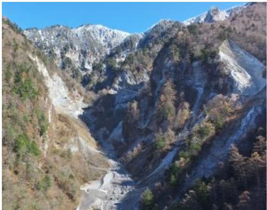
Series of Sabo dams in Shiratani Valley
